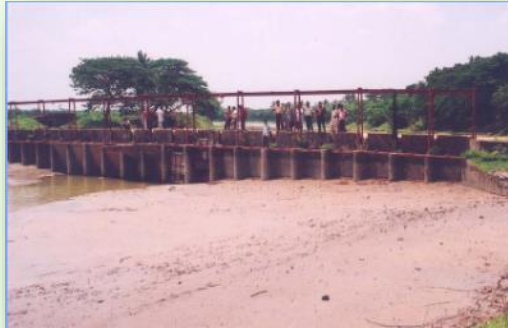
Mega structure on river
